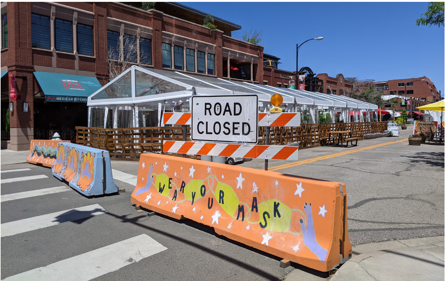
Concrete barriers are a part of the infrastructure upgrades to better serve the need for expanded outdoor dining and walkability areas along Pearl Street in Boulder
